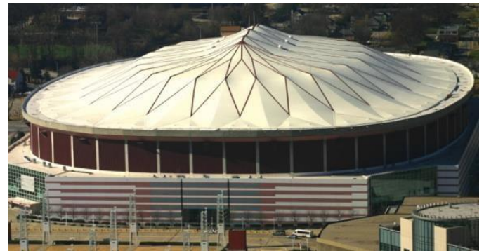
Figure 2: The largest cable dome: Georgia Dome
